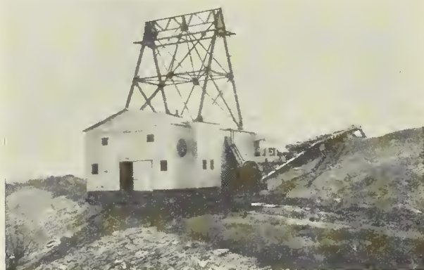
Huge Diesel-powered Dredge Used by Morrison-Knudsen Co. while excavating the three By-passes in Calumet-Sag Canal
